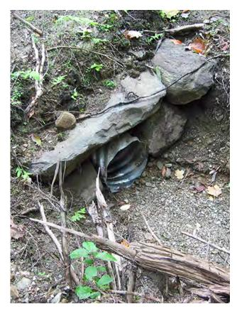
**FIGURE 5.32.** Closed culverts are conduits that move water from one side of the road to the other without it flowing across the road surface. A closed culvert would be used, for example, to move water from a drainage ditch on the up-slope side of a road to the downslope side.
