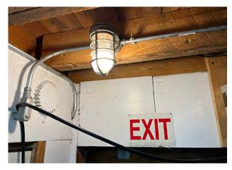
**FIGURE 13.10.** All lights in areas where sap is stored or syrup is processed should be shielded to prevent breakage and glass entering the product.
