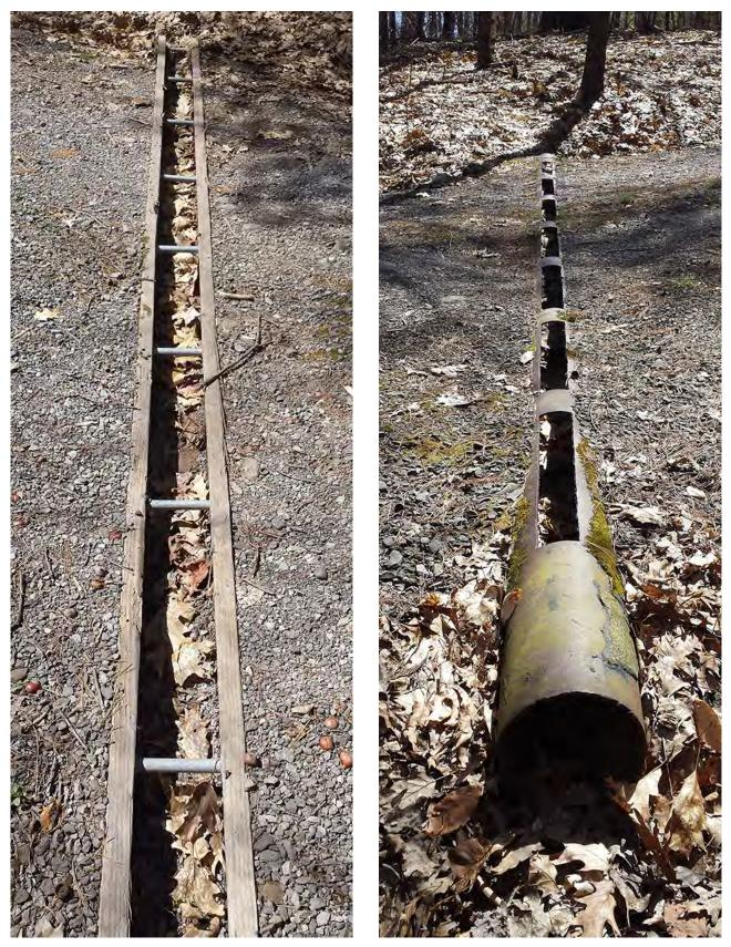
**FIGURE 5.31.** Two examples of open-top culverts. These are installed at a down-slope angle across a road or trail to intercept water and carry it off the road. Culverts require regular maintenance to clear debris.
