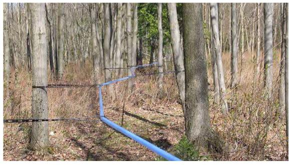
**FIGURE 6.19.** An alternative to standard mainline wire installations, CDL Sugaring Equipment Rapitube<sup>™</sup> allows quick installation with minimal infrastructure. Proper tensioning is required with this product. Frequent side ties or posts should be used to prevent sagging when the pipe is filled with liquid.
