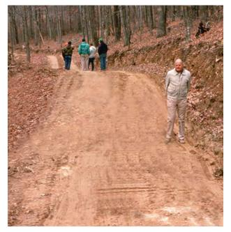
**FIGURE 5.29.** A broad-based dip (foreground) is a low, relatively flat, out-sloped diversion in the roadbed designed to intercept water flowing down the roadbed and drain it to the side, off the road surface. Note the crowned aspect to the roadbed on the rise in the background to facilitate drainage to both sides.
