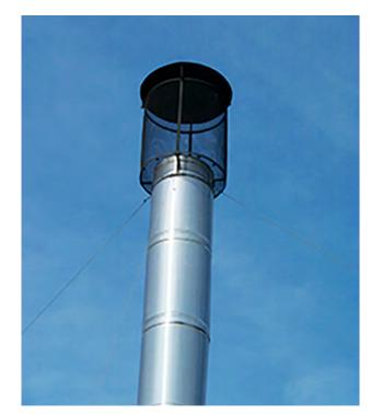
**FIGURE 13.8.** A spark arrester on top of smokestack will help reduce the chance of accidental fires.
