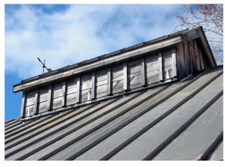
**FIGURE 12.13.** Cupola with pully system to vent steam from sugarhouse.
