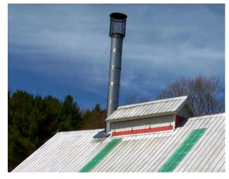
**FIGURE 7.7.** A spark arrester is useful in preventing release of these potential fire starters.
