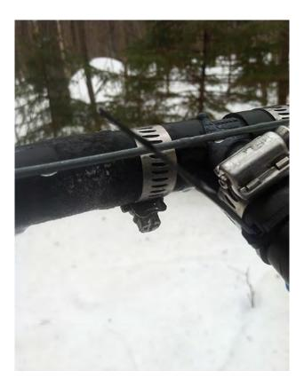
**FIGURE 6.38.** Transitory intermittent ice formation (frost on mainline to the left of the band clamp) caused by microleaks can occur in mainline systems at above freezing temperatures. This leads to loss of vacuum in sections of the woods until the frozen section thaws. These types of leaks are extremely difficult to find and correct.
