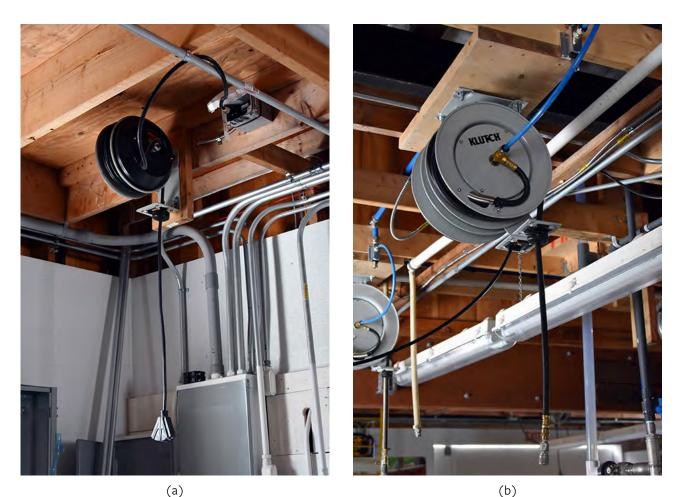
FIGURE 12.8. Electric reel pull-downs (a) and air hose reels (b) offer flexibility in location of equipment.
