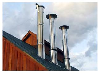
**FIGURE 12.12.** Steam stacks (two rearmost) for venting water vapor from evaporator.
